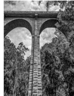
Knapsack Bridge – Emu Plains
