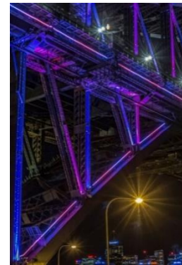
Sydney Harbour Bridge
